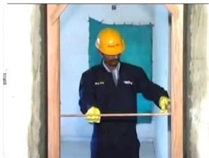
Set the frame true and fix the jigs.
